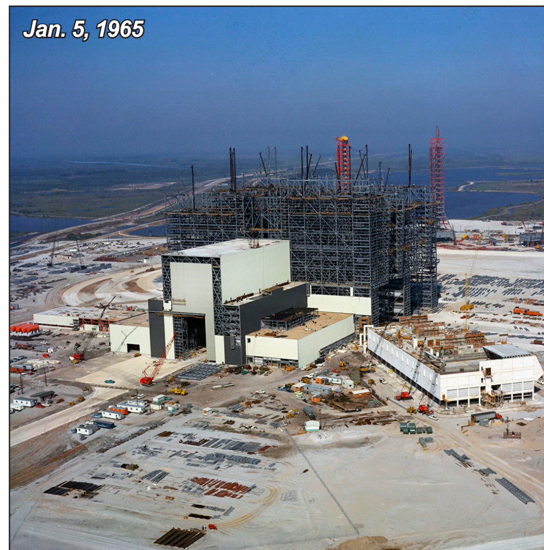
A year and a half after construction start.
