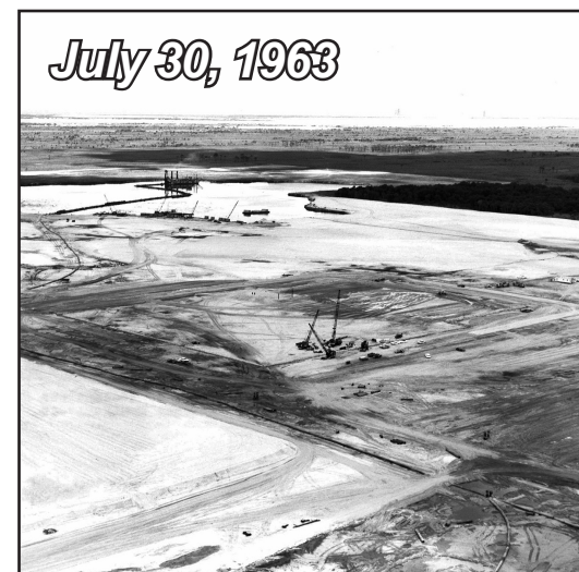
Three large cranes readied for VAB construction.
