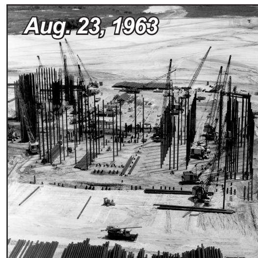
Pile driving in progress.
