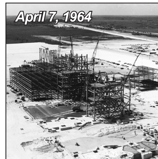
Eight months into construction.
